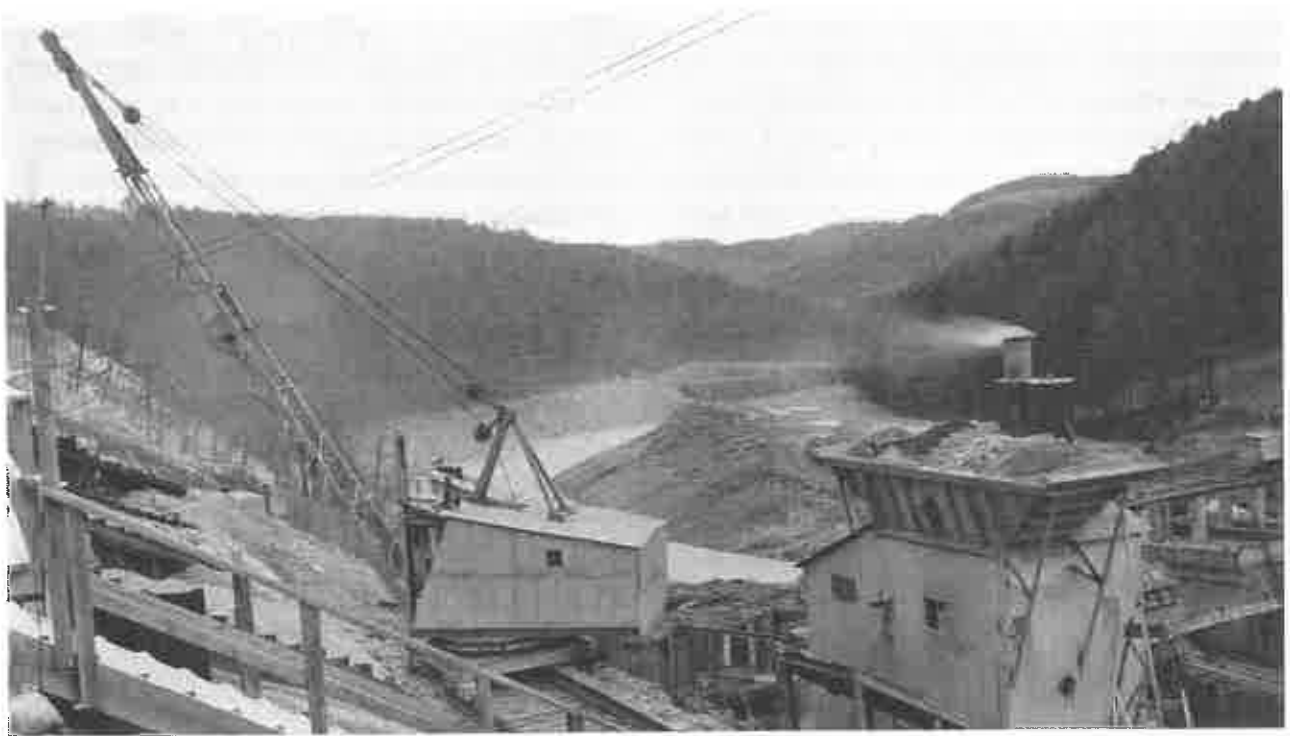
View of plant erected for MIXING CONCRETE at the dam site.
