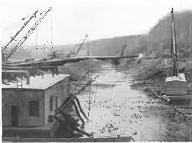
UNWATERING COFFERDAM AND EXCAVATION IN PROGRESS. Pump boat in foreground.
