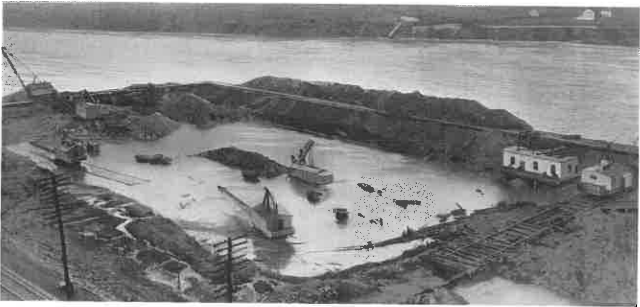
UNWATERING COFFERDAM after flood—EMSWORTH LOCK.
