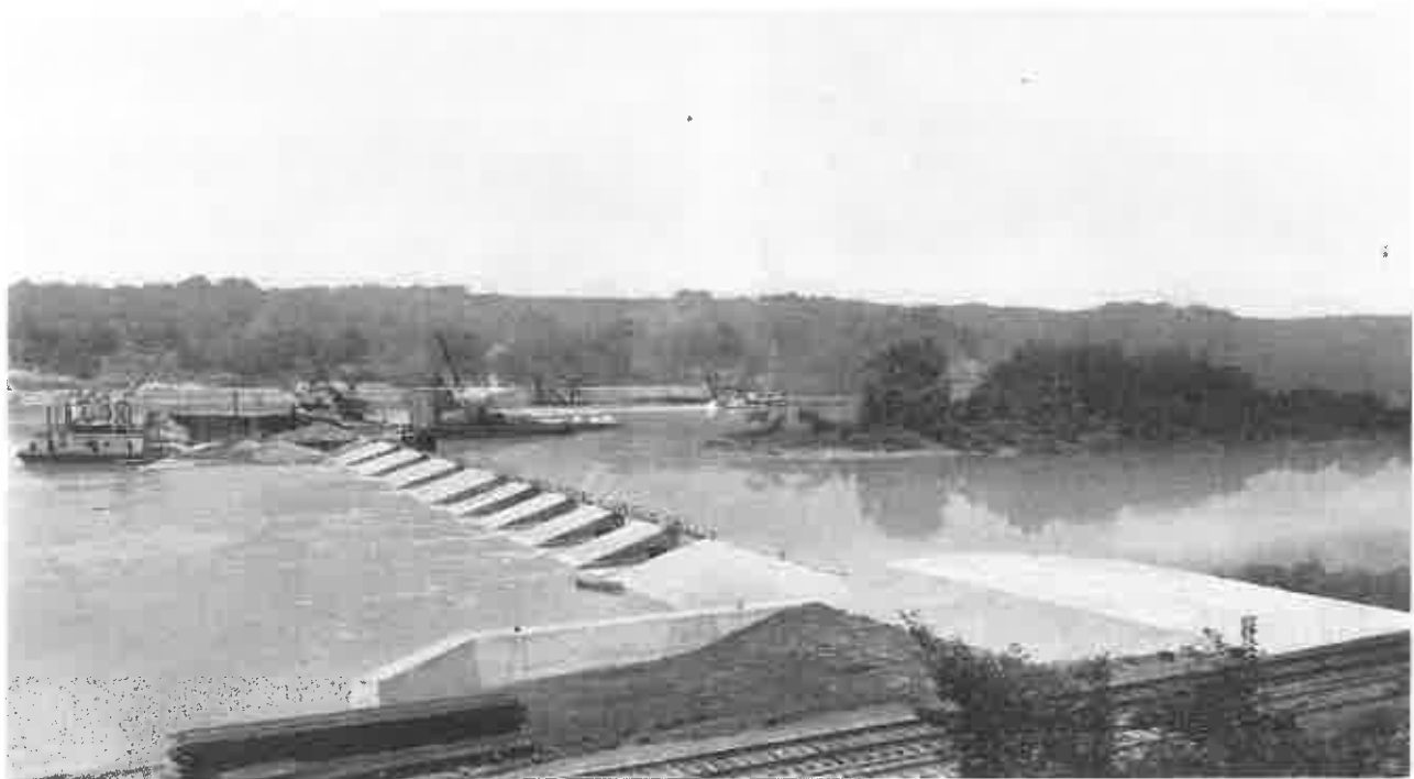
CONCRETING in second cofferdam, DAM No. 6, Allegheny River.
