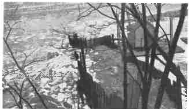
ICE at Upper End of Cofferdam, LOCK No. 7, Allegheny River.
