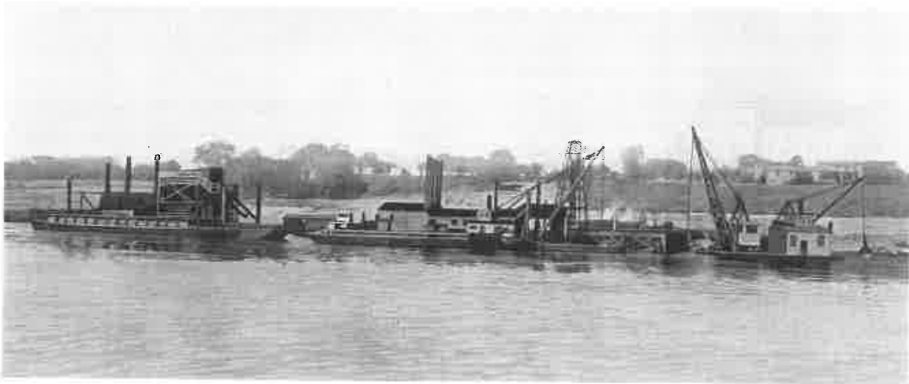
BUILDING COFFERDAM and Excavating for DAM No. 23, Ohio River.
