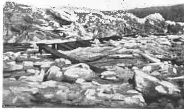
ICE JAM during construction period.
