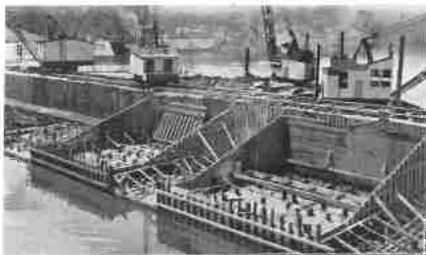
STEEL PILE COFFERDAM at DAM No. 6.
