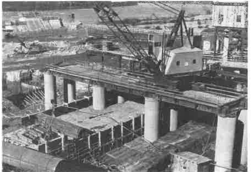
SEVEN CONCRETE-PLACING WHIRLERS operate on the platform supported by CONCRETE COLUMNS 8 feet in diameter. The columns are ultimately incorporated into the dam.
