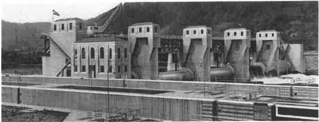
The ROLLER GATE RECESSES AND OPERATORS HOUSES here reveal the scheme of hoisting gates from one end only and the seals at the faces of the piers.
