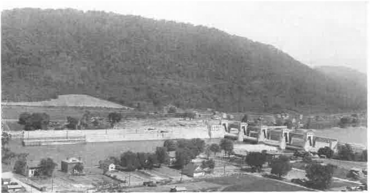
A GENERAL VIEW OF THE LOCKS AND DAM showing flap gate with flap raised.
