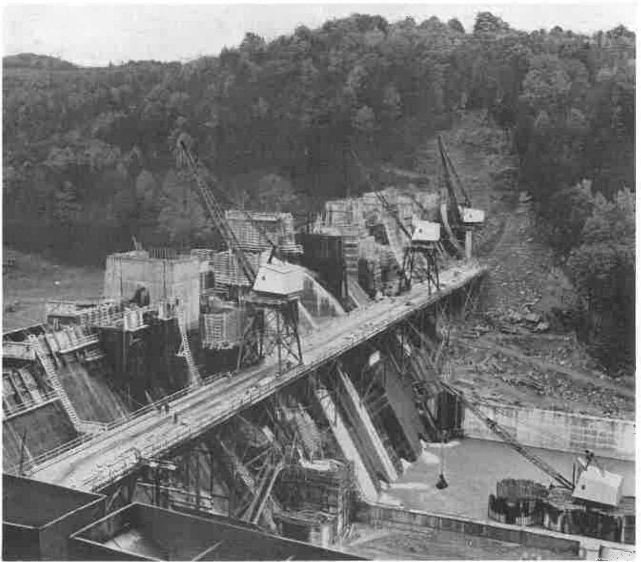
DRAVO WHIRLERS, mounted on GANTRIES on the concrete dinkey track bridge, dominate the scene as Mahoning Dam rises.
