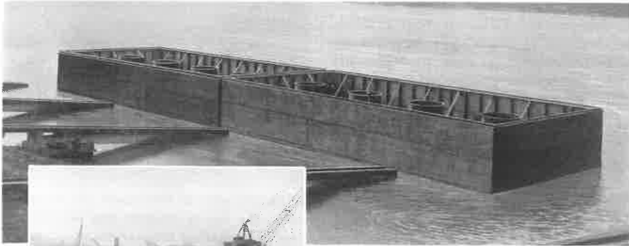
STEEL FLOATING CAISSONS launched at our Neville Island Yards for DAM No. 32, Ohio River.
