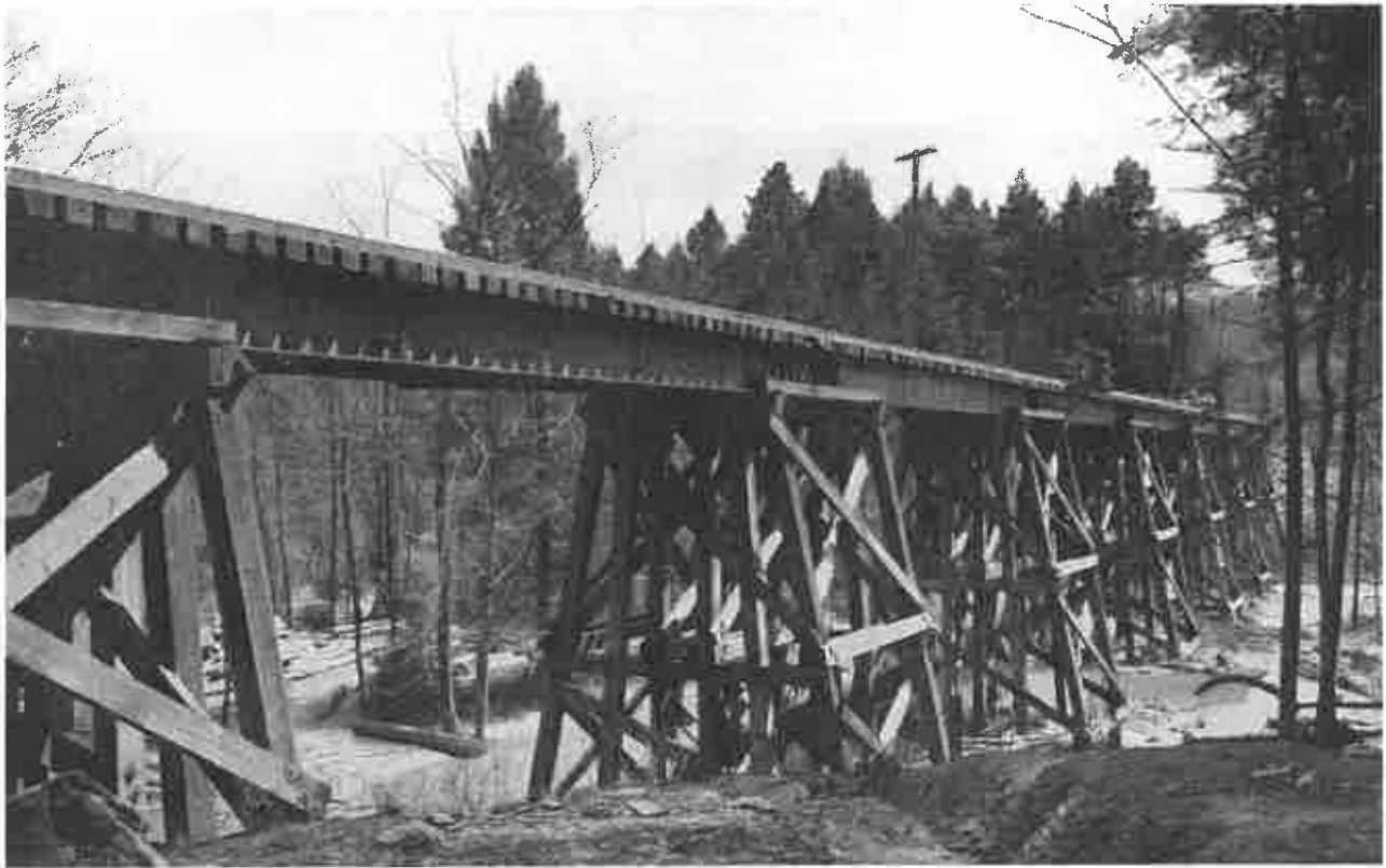
To move aggregates to the dam site, a 3.8 MILE SPUR TRACK was constructed. Here a section of track crosses a ravine over a DRAVO DESIGNED AND CONSTRUCTED TRESTLE.
