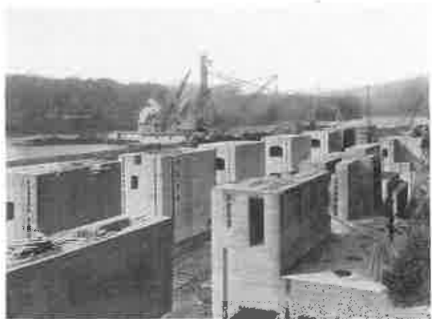
WALLS BEING BUILT IN ALTERNATE MONOLITHS. Floating mixer plant in background.
