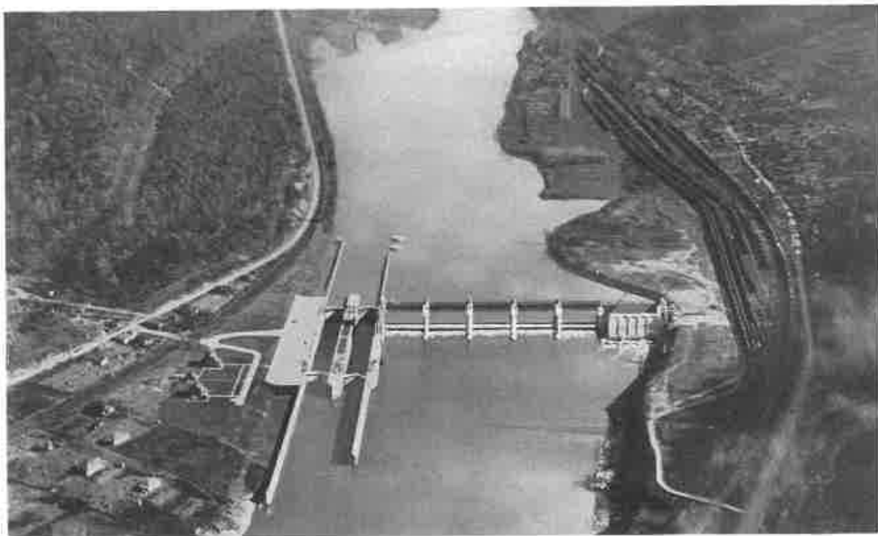
LONDON LOCK AND DAM performs a vital function in the Industrial Development of Kanawha Valley.
