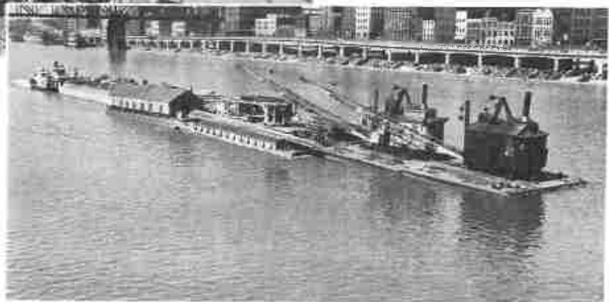
Derrick Boats, Power and Shop Boat, Barges of Equipment and Materials and small Towboats enroute to start new construction operations.
