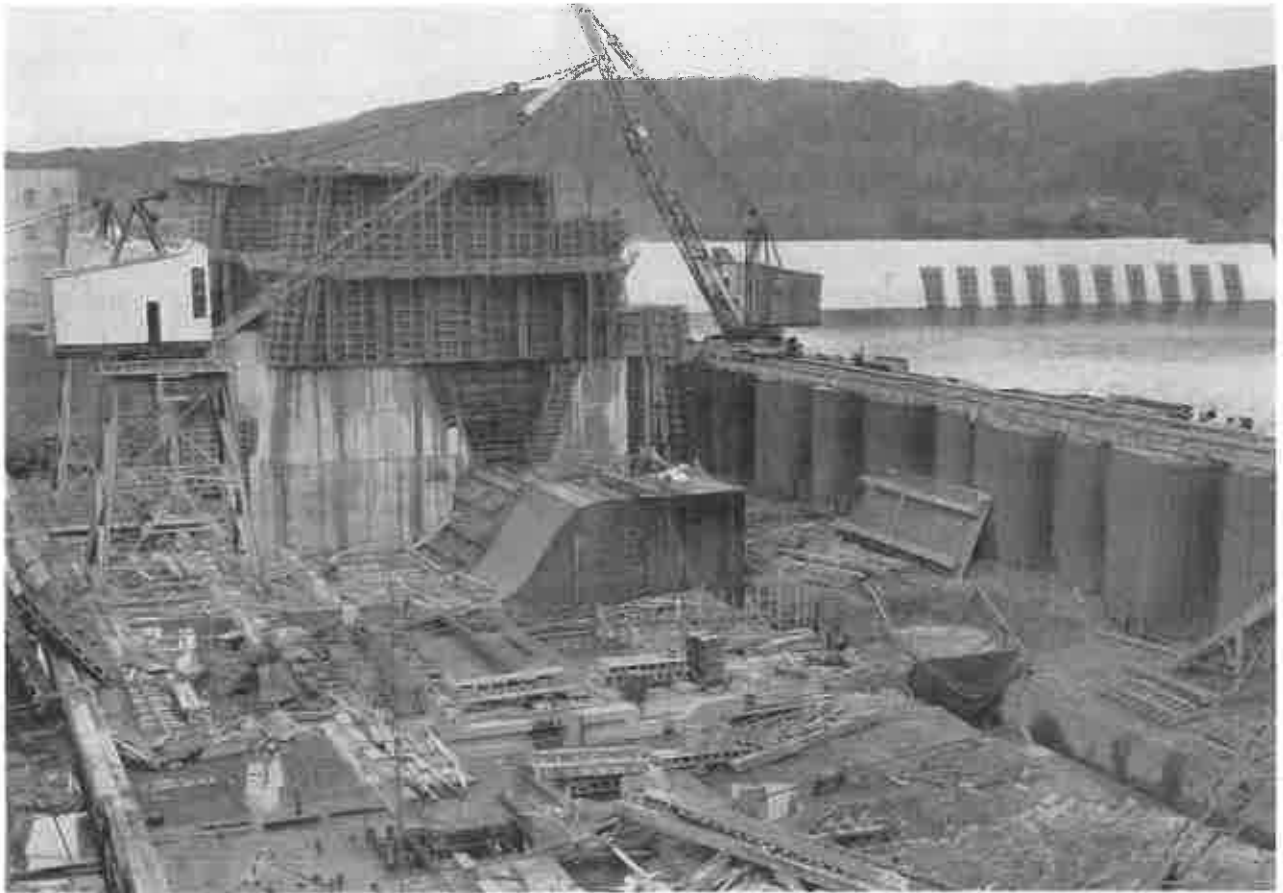
The PIER AND SILL CONSTRUCTION was greatly facilitated on this project by the use of DRAVO GANTRY WHIRLERS.
