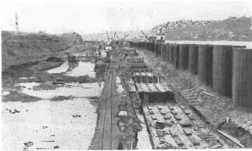
With sixteen acre COFFERDAM COMPLETE AND WORK in progress.
