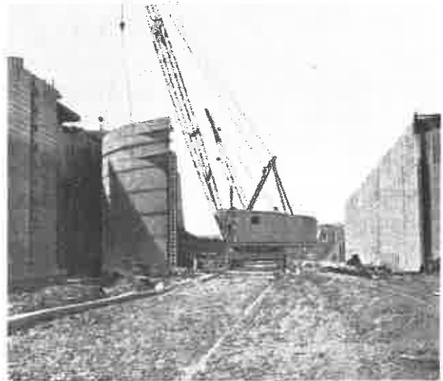
Erection of LOCK GATES.
