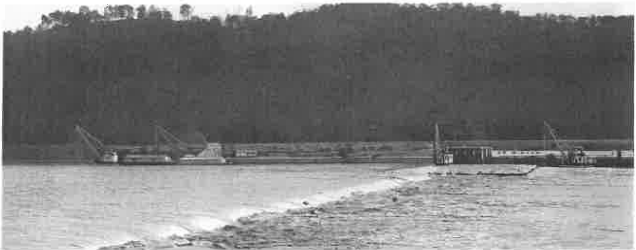
Ohio River in flood at DASHIELDS DAM with WATER OVERTOPPING COFFERDAM.
