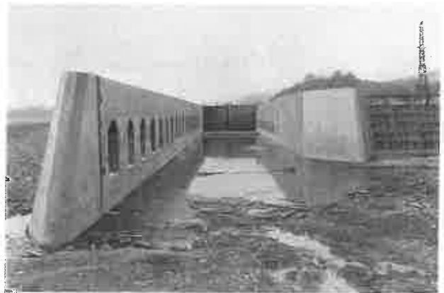
View from upper end of EMSWORTH LOCK.
