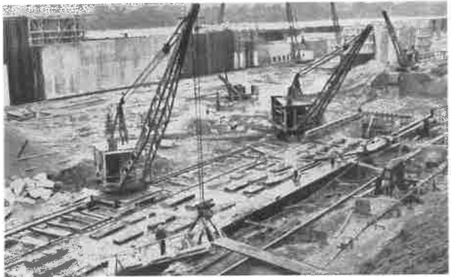
General view of LOCK CONSTRUCTION featuring the application of WELL POINTS in foreground.
