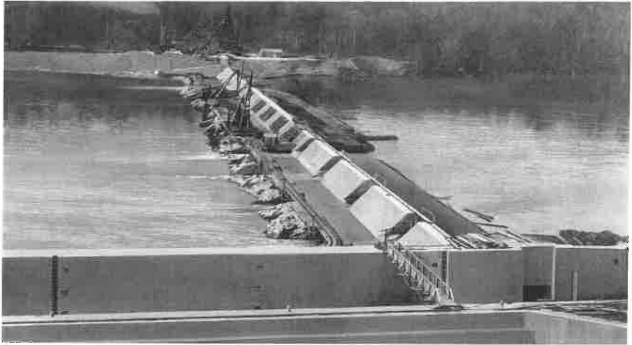
LOCK AND DAM No. 14, Black Warrior River.
