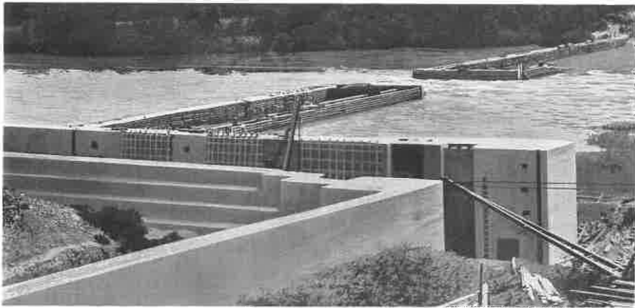
LOCK AND DAM No. 15, Black Warrior River.
