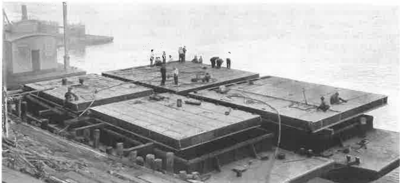
GATES FOR LOCK No. 7, Monongahela River being assembled on Barges at our Neville Island plant. These gates of the mitring type, as well as the fixed metal work and the butterfly valves in connection with the project, were furnished by our Engineering Works Division.
