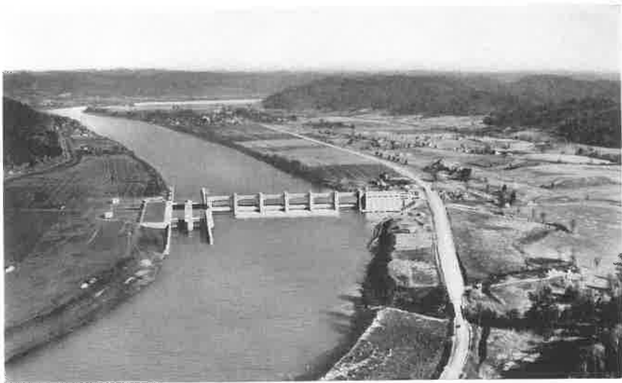
The INDEPENDENT OPERATION OF EACH ROLLER GATE is revealed in this view of the completed Winfield Lock and Dam.
