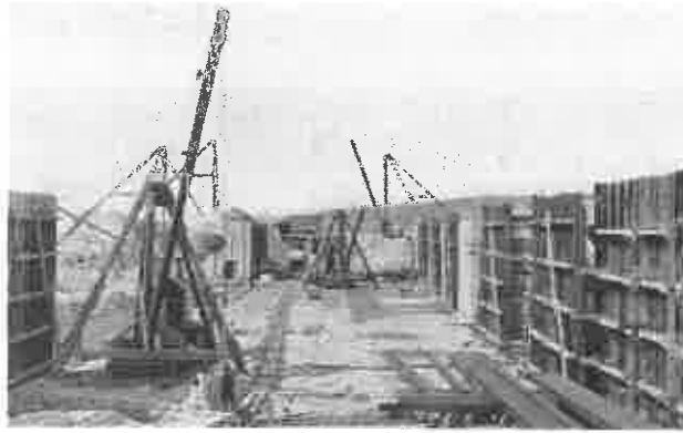
General View of operations.
