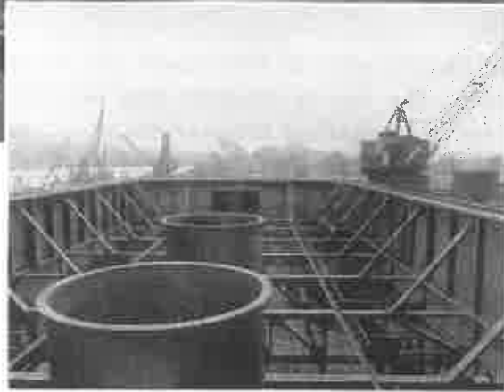
Interior View of STEEL FLOATING CAISSON.
