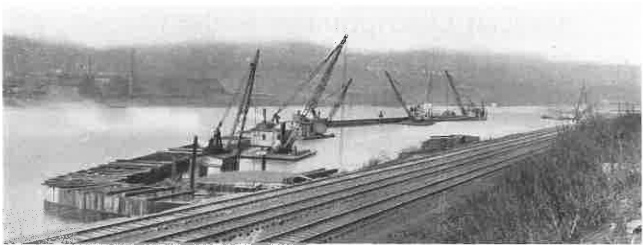
BUILDING STEEL PILE COFFERDAM for LOCK No. 4, Monongahela River with Dravo built Whirler Boats.
