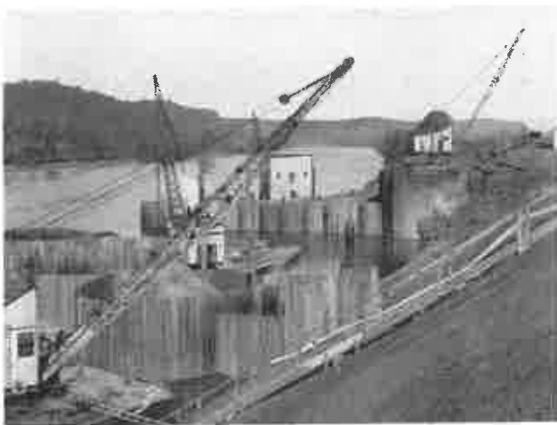
A battery of DRAVO WHIRLER DERRICK BOATS busily engaged on cellular cofferdam construction.
