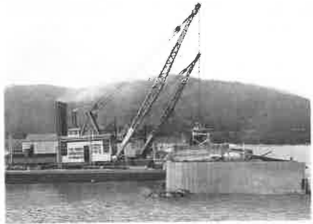
SINKING CAISSONS at DAM No. 32, Ohio River.
