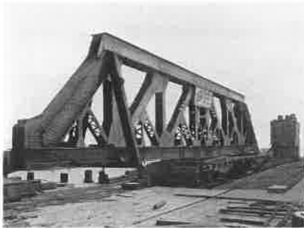
THE MAIN TRUSS—88'8" long, 13'9" high, weighing 45 tons.
