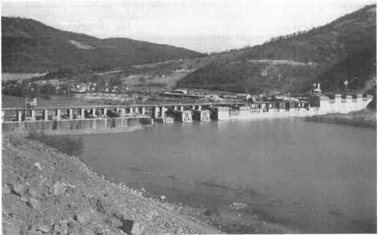
UPRIVER VIEW OF BLUESTONE DAM rising out of the New River just south of Hinton, W. Virginia. When completed the dam will impound 631,000 acre-feet of water, creating a reservoir approximately 35 miles long.
