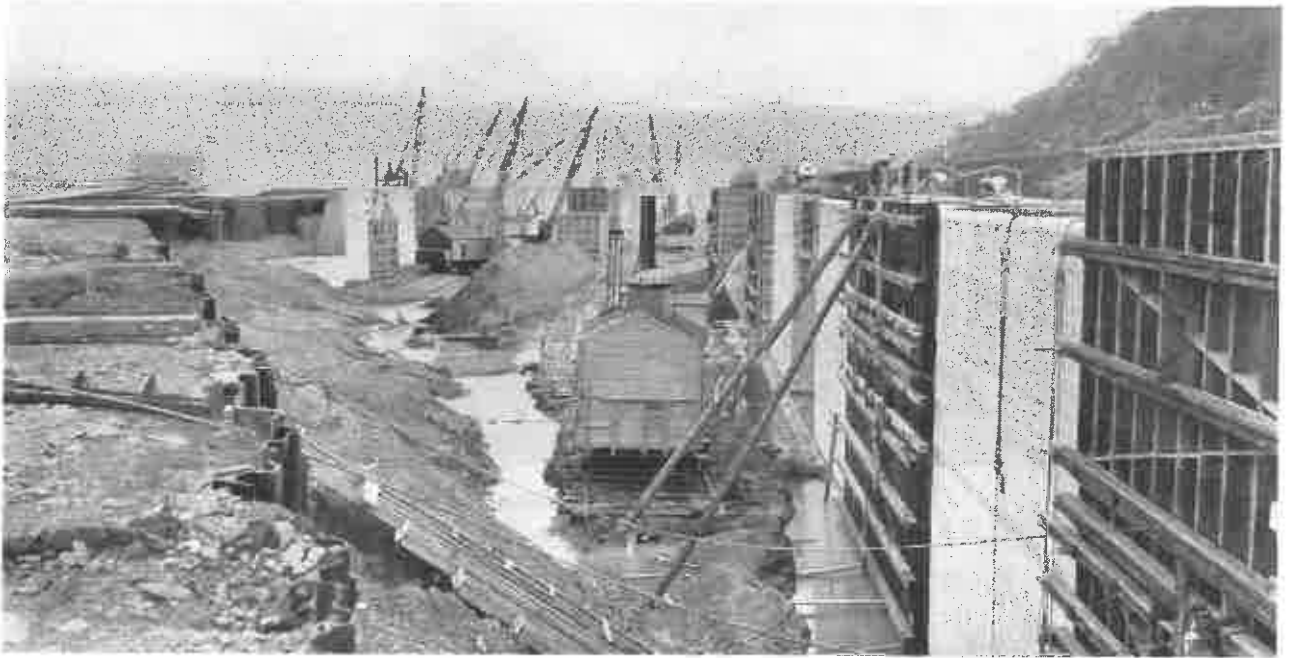
General View of Operations at LOCK No. 4, Monongahela River. Note Steel Pile Cofferdam at left.
