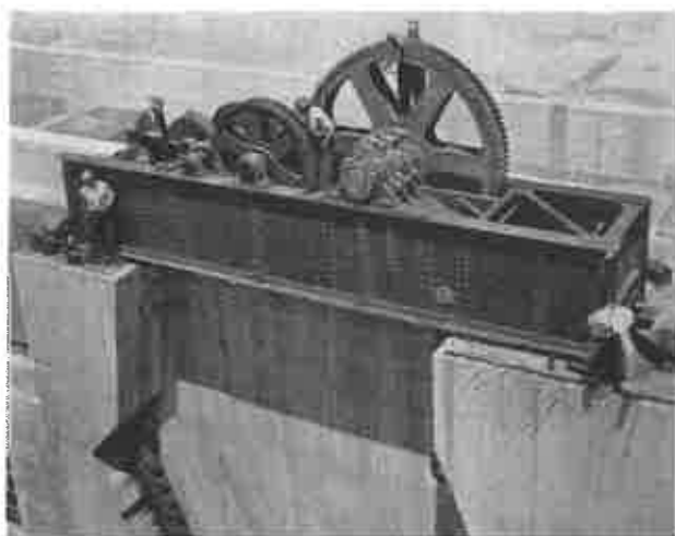
Erecting ROLLER GATE HOIST at Gallipolis Dam.
