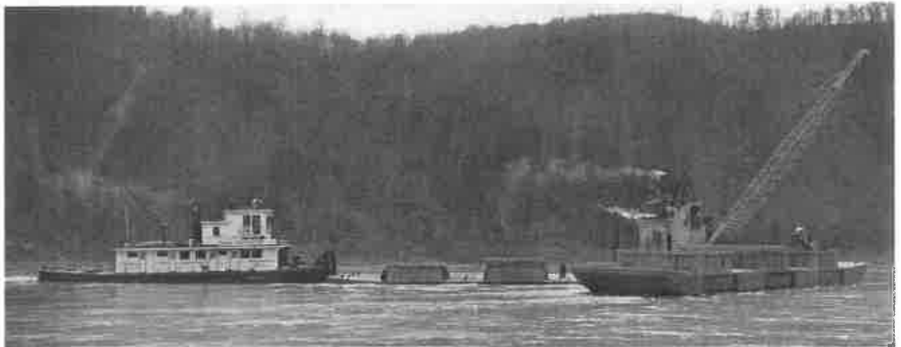
DREDGING OPERATION IN THE ALLEGHENY RIVER. Concrete aggregate for Mahoning Dam was prepared from this dredged material.
