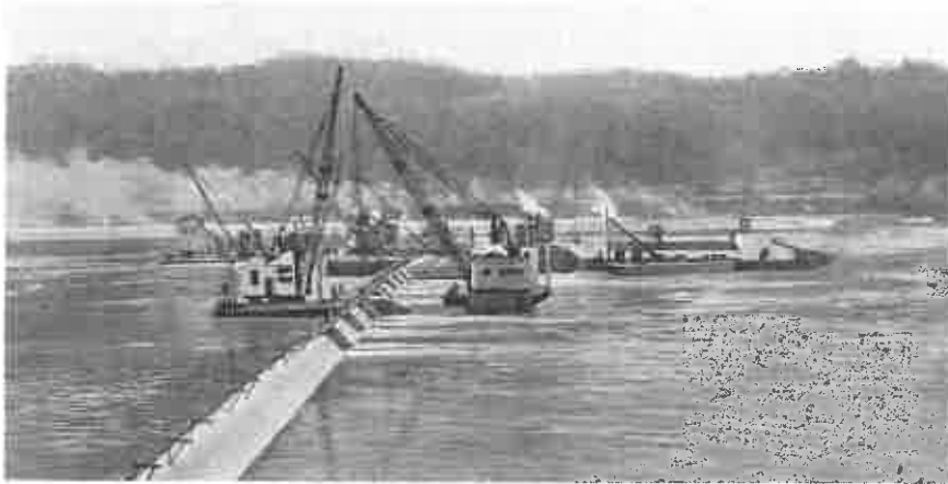
PLANT AND EQUIPMENT working at DASHIELDS DAM.
