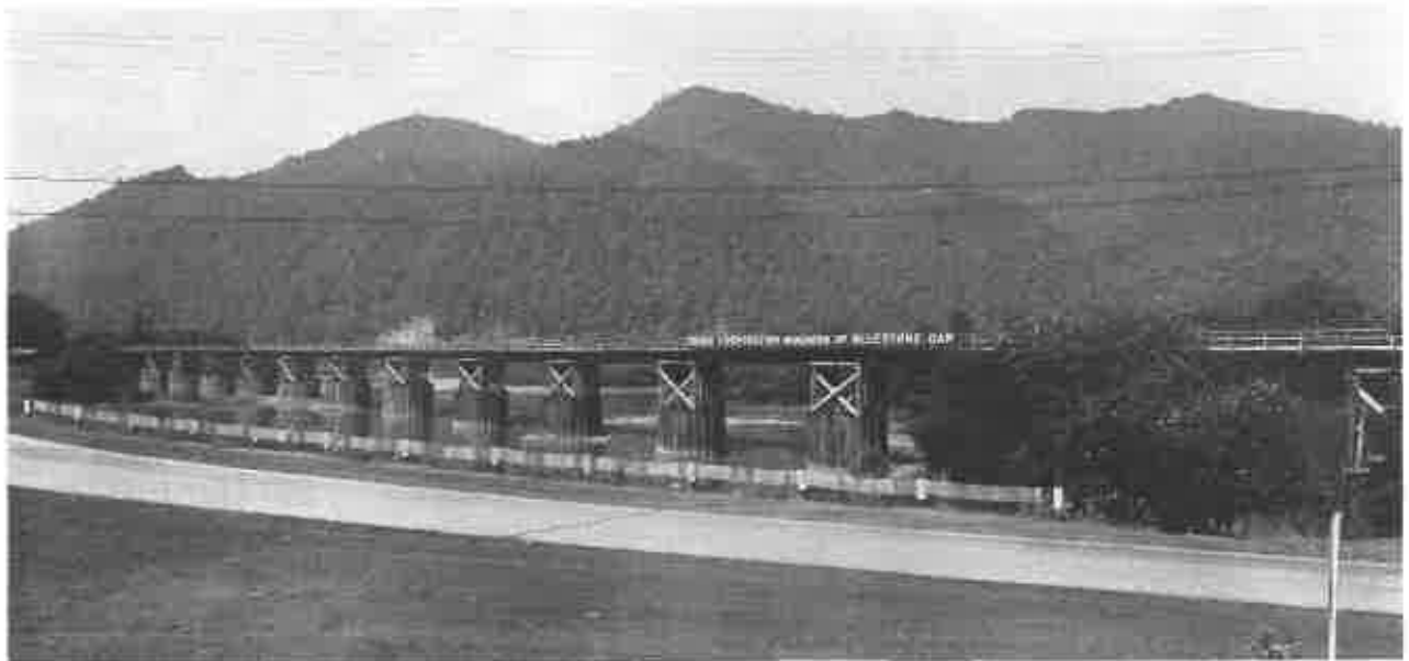
RAILROAD BRIDGE constructed by Dravo to facilitate movement of material to dam site.
