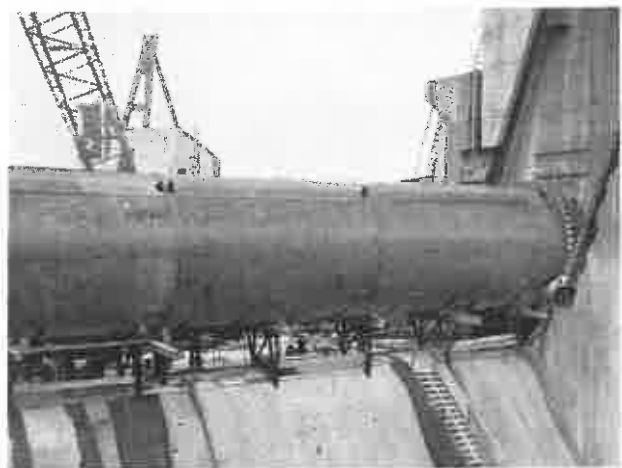
ROLLER GATE erection showing clearly the Pier Recess and the supporting Sill.
