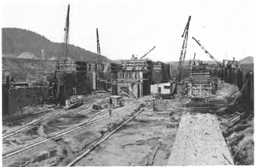
A general view of LOCK CONSTRUCTION featuring the extensive HEAVY EQUIPMENT required.
