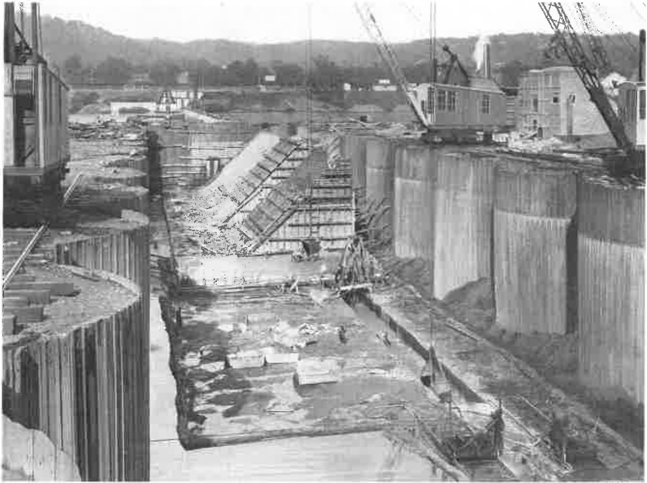
CONCRETING AND EXCAVATING for DASHIELDS DAM. Note verticality of steel piling.
