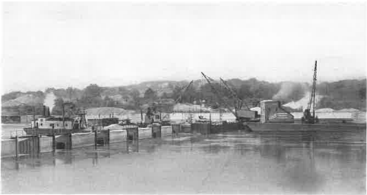
General View of operations at DAM No. 6, Allegheny River.
