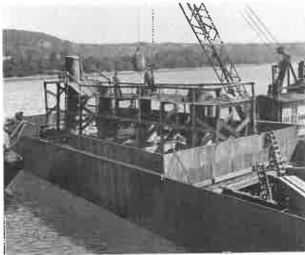
EXCAVATING CAISSON through Air Locks, DAM No. 32, Ohio River.
