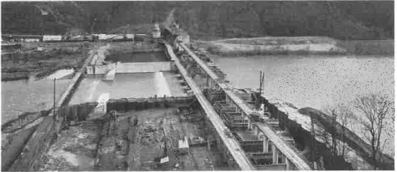
3-YARD BUCKETS OF CONCRETE move along the tracks in cars to the pouring site where they are dumped by DRAVO WHIRLERS. Approximately 1,000,000 yards of concrete will go into Bluestone Dam.
