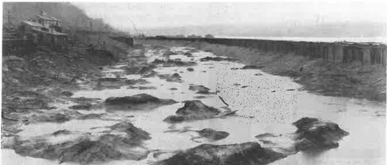
UNWATERING COFFERDAM for LOCK No. 4.
